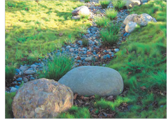
Landscape bioswales reduce stormwater runoff
